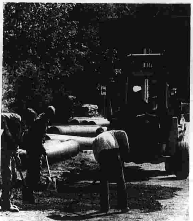
Members of the Town of Manchester's Water Department did a little road work Tuesday after they completed preparation work for today's replacement of part of a wooden line in Glastonbury residents serviced by the line to continue to receive water while the line replacement is done. (Herald photo by Chastain)
